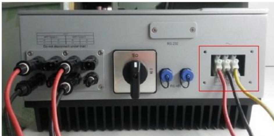
Fig.11 AC cables wiring
